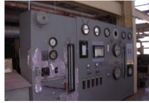
1. Panel, Switchgear, Turbine and Generator Control
