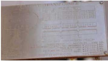
ABL-609 Abilene Plant Unit 4 Unit Auxiliary Transformer (434-2) Out of service and drained 3/25/2003, Moloney Transformer Serial # 855771, Type SPL, 3 phase, 60 cycle, 750 KVA continuous 55c rise, High Voltage 13200, Low Voltage 480, % Impedance 5.45, Gal Oil 455 gallons, Mfg. Date 4/30/48, Un-tanking Height 15 ft. 6 in., Un-tanking weight 4600 lbs., Tank & fittings 3300 lbs., Oil weight 3425 lbs., Total weight 11325 lbs.
