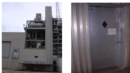
OAK-430 1. Elevator, Boiler Access
