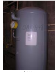
OAK-448 1. Tank, Air receiver, Control Air Receiver
