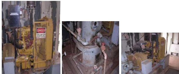
OAK-457 1. Pump, Firewater, Vertical
