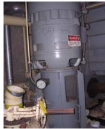
OAK-446 1, Pump, Centrifugal Number and Type: Two 16QEC-7 stage, vertical pit mounted, removable rotor type centrifugal pumps, Motor: 125hp, 1180rpm, 2300 volt open, dripproof motor, Performance Data: capacity: 950gpm, Net developed Head: 350ft, Shutoff Head: 395ft, Efficiency: 77%, Bhp: 109, Pump Data: Mfr: Worthington Corporation, Gpm: 950, RPM: 1180, Head Feet: 375, Driver HP: 125, SN: 1587903, with motor, electric, Mfr: Westinghouse, HP: 125, Phase: 3, Cycle: 60, Frame: 580 PH, Design: B, Cont. Speed, 40°C, Volts: 2300, Amps: 28.3, RPM: 1180, KVA Code: E, Style No.: 19N6935, SN: 2S-60
