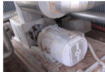
OAK-429 1. Pump and Motor Assembly
