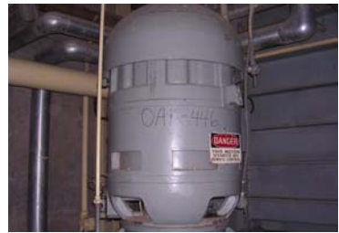
OAK-446 1, Pump, Centrifugal Number and Type: Two 16QEC-7 stage, vertical pit mounted, removable rotor type centrifugal pumps, Motor: 125hp, 1180rpm, 2300 volt open, dripproof motor, Performance Data: capacity: 950gpm, Net developed Head: 350ft, Shutoff Head: 395ft, Efficiency: 77%, Bhp: 109, Pump Data: Mfr: Worthington Corporation, Gpm: 950, RPM: 1180, Head Feet: 375, Driver HP: 125, SN: 1587903, with motor, electric, Mfr: Westinghouse, HP: 125, Phase: 3, Cycle: 60, Frame: 580 PH, Design: B, Cont. Speed, 40°C, Volts: 2300, Amps: 28.3, RPM: 1180, KVA Code: E, Style No.: 19N6935, SN: 2S-60
